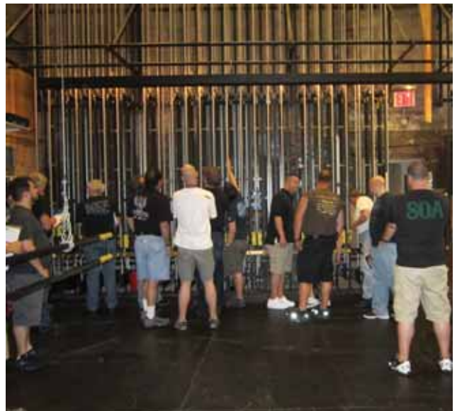
Rigging System Inspection
