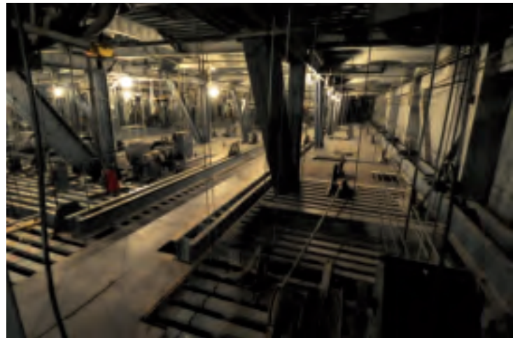
Spot Grid Iron: 113 feet above the deck
